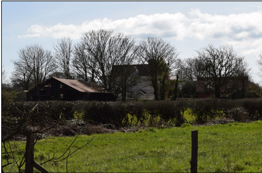
Plate 24: View of northern part of Peel Farm, looking south-east from Newgate Lane (zoom image)
