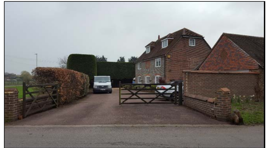
Plate 25: Carriston Cottage, looking south
